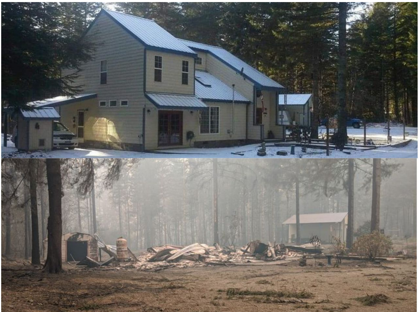
Fred Trummell's home in Lyons before the Beachie Creek fire (above) and after. Courtesy/Fred Trummell
